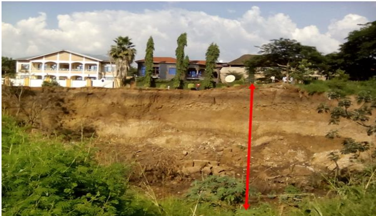
Picture 5 : Example of threat of destruction of Kigobe houses
