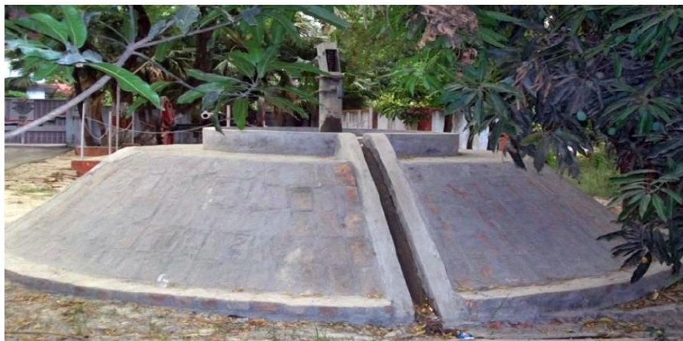
Figure 36 : Anti-flood hand pump
