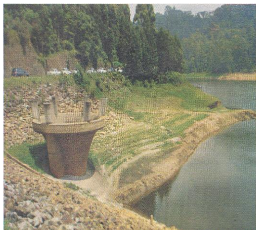
Picture 3 : Dam level of Rwegura CHE in 2008
